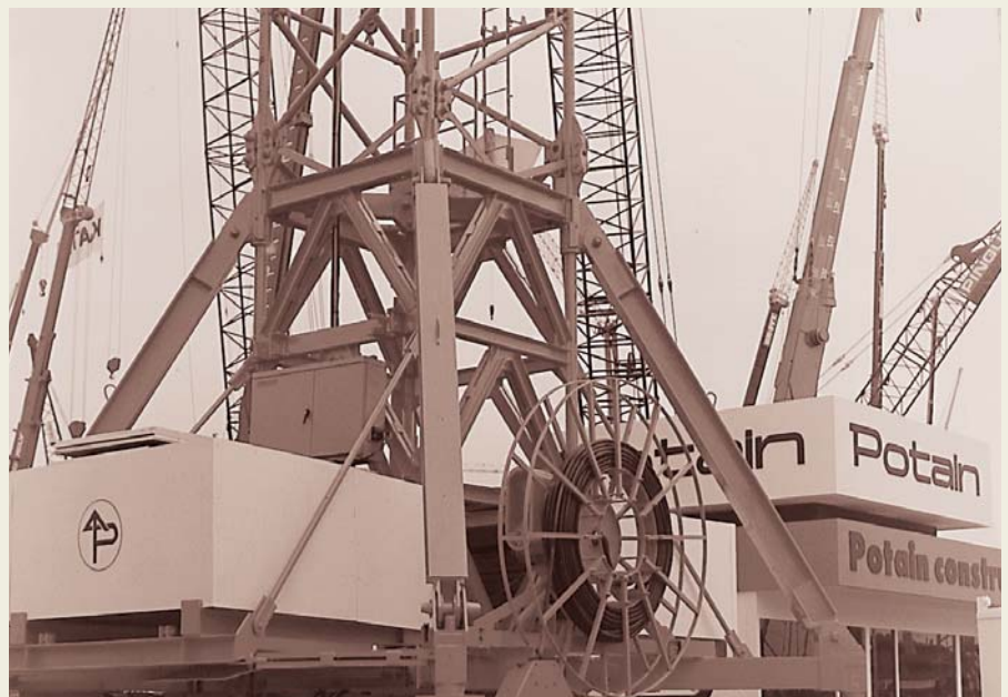
Potain tower crane - 1966.
