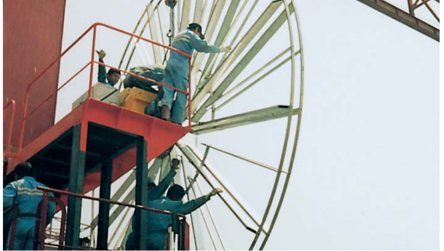
One of our drums during erection in a harbour application in Singapore.
